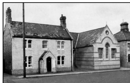
Broad Street school, with the master's house on the left and schoolroom on the right. There are further rooms behind.
